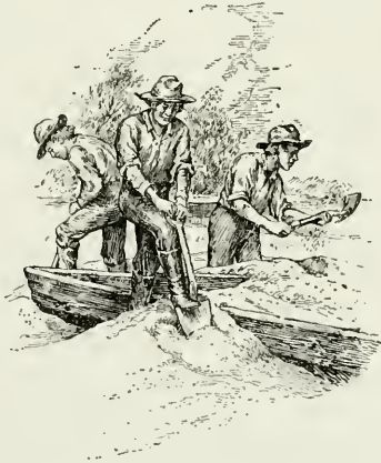
Digging out the scow.
